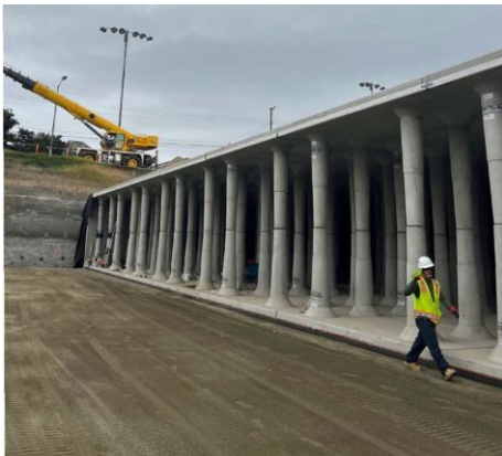
Subsurface Infiltration Gallery
