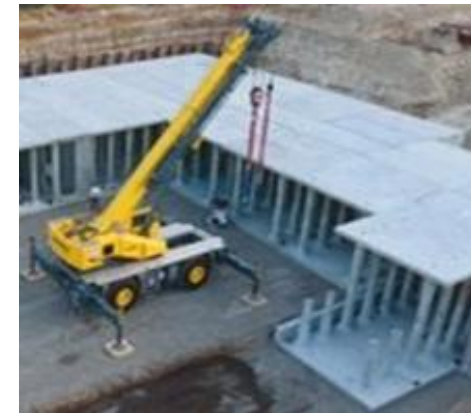
Subsurface Infiltration Gallery
