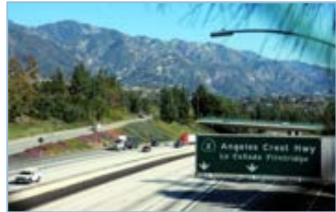
Foothill Freeway approaching SR-2
