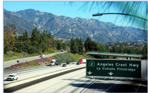
Foothill Freeway approaching SR-2
