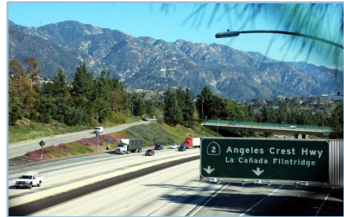
Foothill Freeway approaching SR-2
