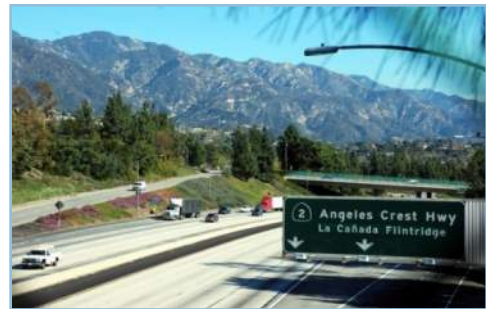
Foothill Freeway approaching SR-2
